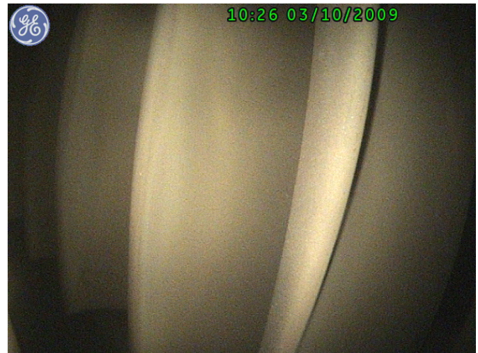
Figure 2: Typical Stage-2 blade after 5,000 (new)/12,200 (refurbished) hours of operation
